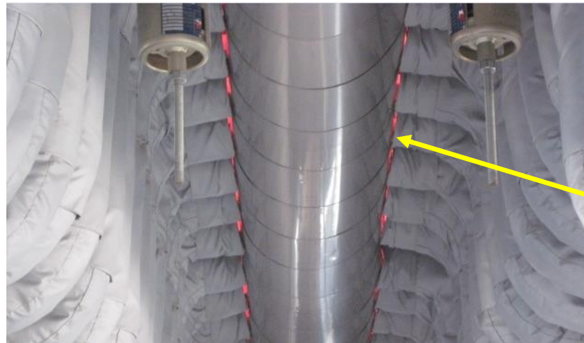
Spring Hanger bottomed out (no load)
