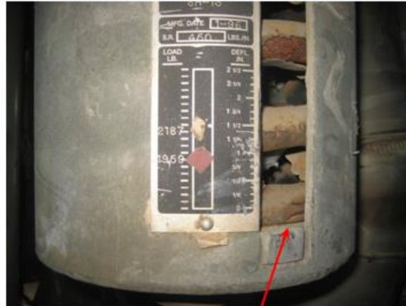
Spring Hanger bottomed out (no load)
